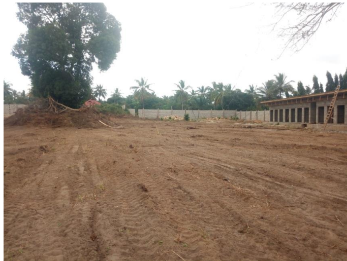
Figure 4: Bus stand and commercial building structures both under construction
